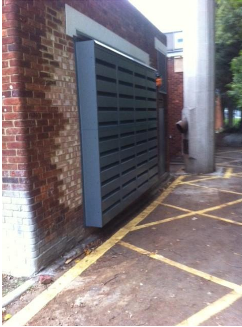
Acoustic louvre to back of plant room
